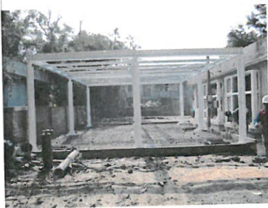
基礎開挖/鋼結構組立 Foundation excavation / Steel structure assembling
