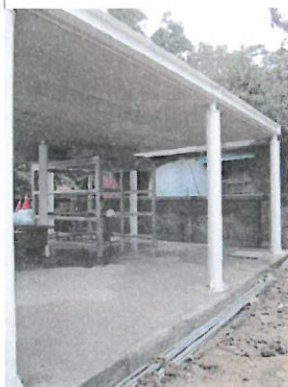
封車棚天花 Ceiling installation
