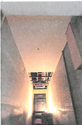
封天花板 Ceiling installation
