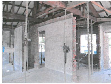
結構內牆拆除 Interior structure demolition
