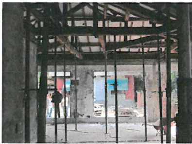
假設工程 Suppose supporting
