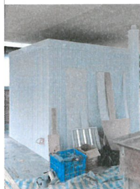
車棚機房建置 Engine room building
