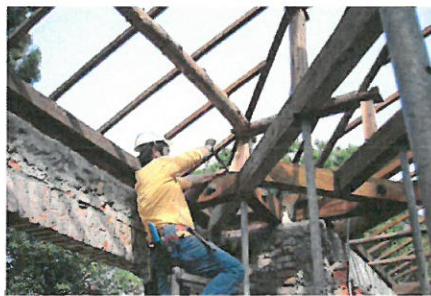
屋頂椽木更換修補 Replacing wooden roof rafters
