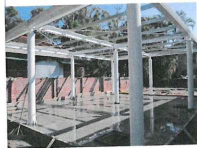
地坪灌漿 Floor grouting
